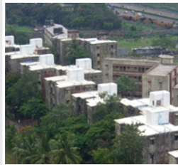
Railway Quarters, Ghatkopar Mumbai
