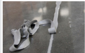
Shaving excess UREGEL off
