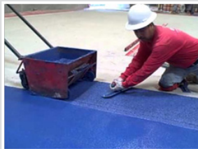
Preparation with URECRETE SC
