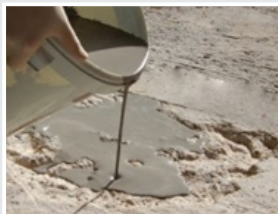
INCRETE PMR Priming stage 2
