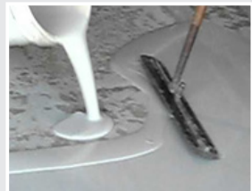
INCRETE PMR Placing stage 3
