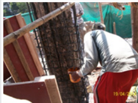
TECHNORUST on exposed rebar
