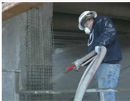
PCI 200 additive in sprayed mortar
