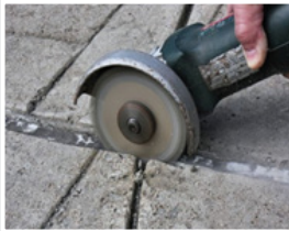
Saw cut before placing SILIGEL
