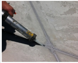
Placing SILIGEL for concrete joints
