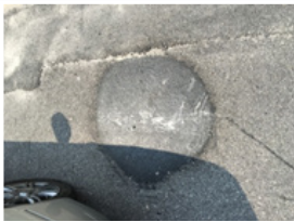
Trench Patching Seremban, Malaysia
