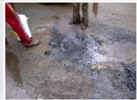
Water filled Pothole Repair PWD, Pune, India
