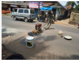
Utility Patch Repair Mangalore, India
