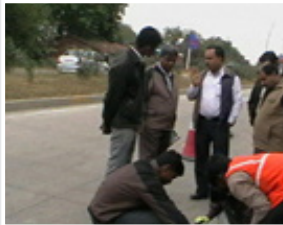
INCRETE PMR Priming stage 2
