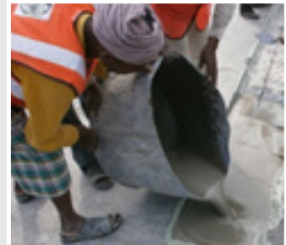
INCRETE PMR Placing stage 3
