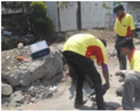
INCRETE PMR Breaking stage 1
