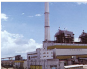
Reliance Power Plant, Dhanu
