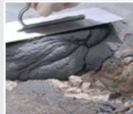
Concrete floor patching
