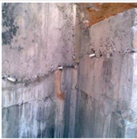
INCAP GROUT for retaining wall
