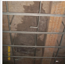
Before INCAP GROUT application
