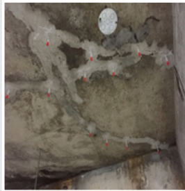
INCAP GROUT for ceiling
