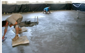
Base Preparation with Screed
