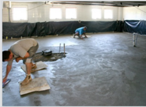
Base Preparation with Screed
