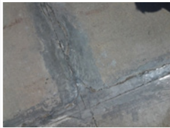
Floor joints filled with EPIGEL
