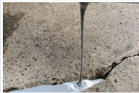
Semi rigid cracks filled with EPIGEL
