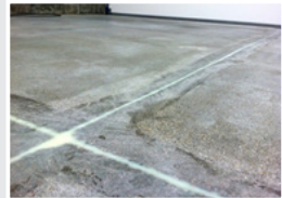
Floor joints with EPIGEL
